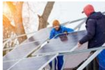
install a system
